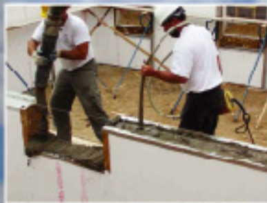
Concrete Consolidation
